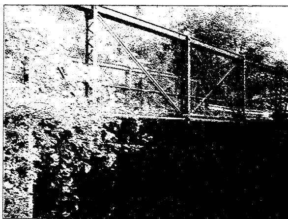
Photo by Marsha Johnson Chartrand The Furnace Street bridge has been closed for more than 10 years. But recent traffic concerns have prompted the village to take a second look at reopening the structure to vehicle traffic.
