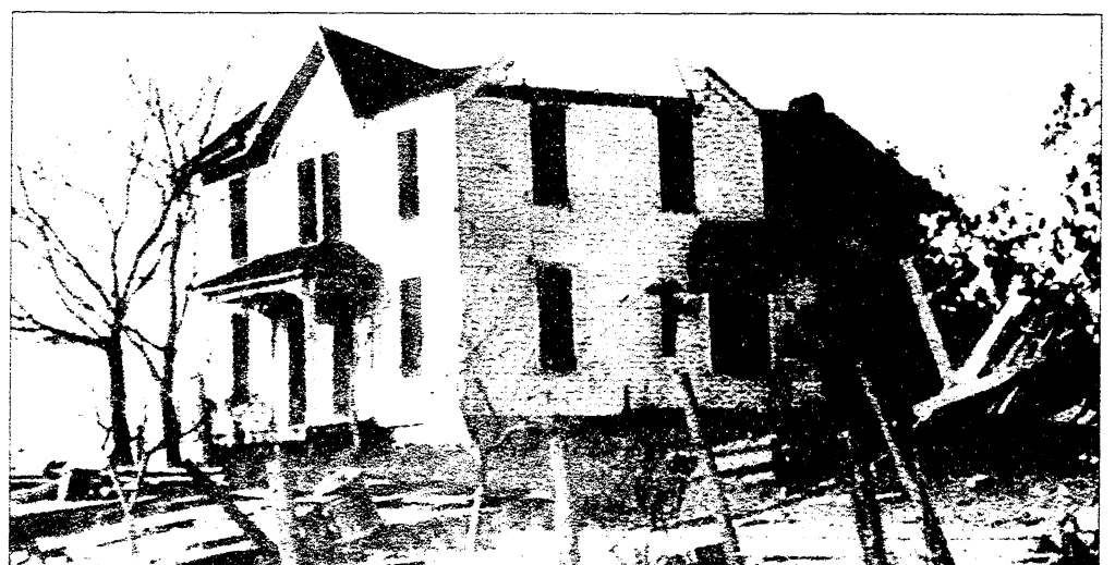
The Old Zion Parsonage is pictured here after a June 6, 1917 cyclone tore the roof off the house. The storm also destroyed the old church's bell tower and roof as well as several nearby homes, according to longtime neighbor and Zion Lutheran member Norm Wenk.
