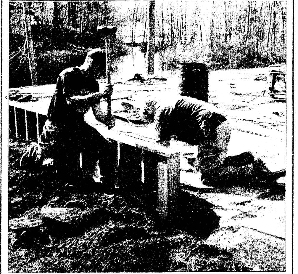
Monday brought sunny skies and 58-degree temperatures, perfect for mounting a floor joist on this property at 320 Riverside Drive. Pictured, from left, are Nathan Parker and Paul Messer of Carver Construction Company of Ann Arbor. Together with Jerry Seger (not pictured), they tore down the condemned former gas station and auto repair shop last week to make way for a two-story duplex to be built on the existing foundation. Asked if the crew planned to keep working despite a forecast for snow, Messer replied, "Don't put it past us. We'll move the snow aside and keep working."
