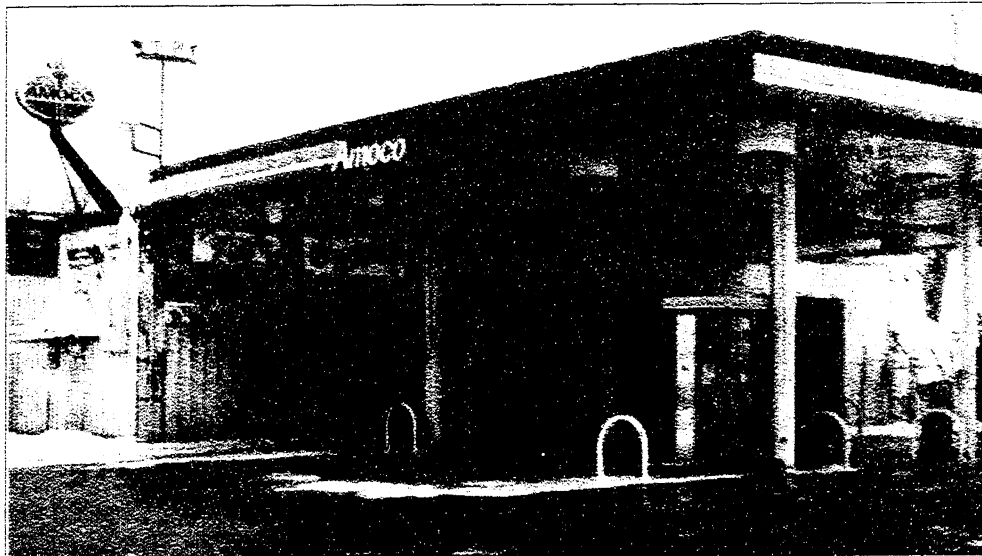
G.E. Wacker, Inc., in Sharon Township, will soon be home to the first biodiesel fuel pump in the state of Michigan. The fuel, made from vegetable oils, is more efficient and cleaner than regular diesel fuel.
