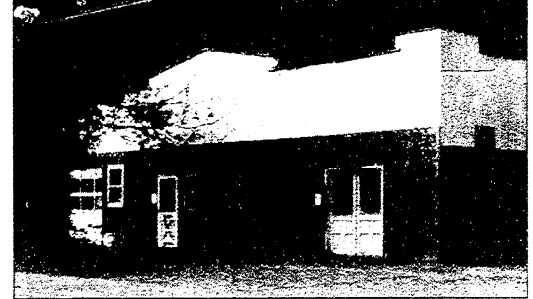
This building, once a gas station and automobile repair shop, will be renovated by Carver Construction and made into duplex townhouses.
