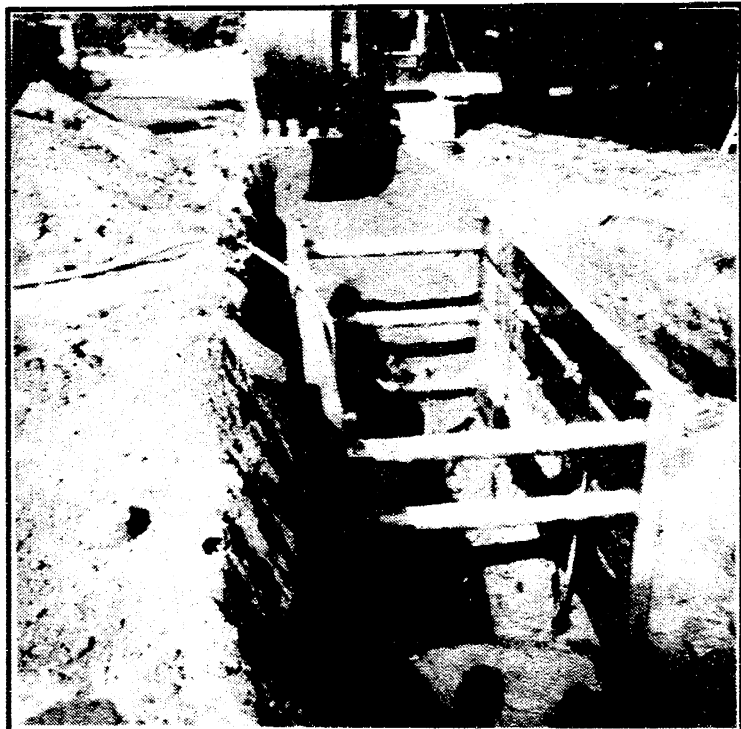
Sewer Problems: Steel Trench Box in Hole on East Main Street - see story on page 13
