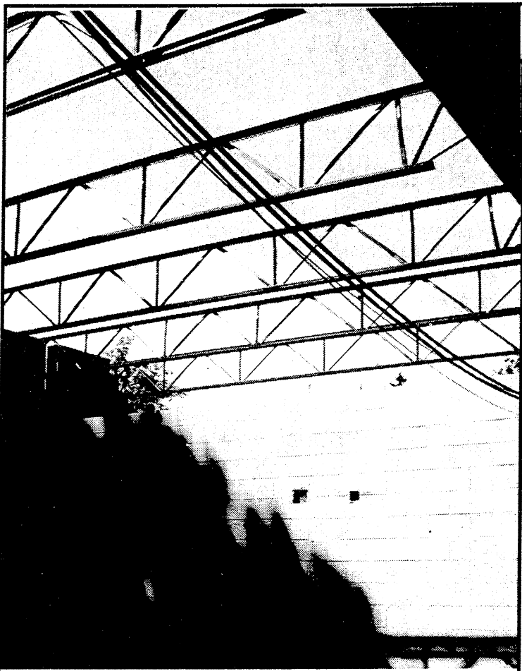
Construction at the Middle School included the installation of these roof trusses.
