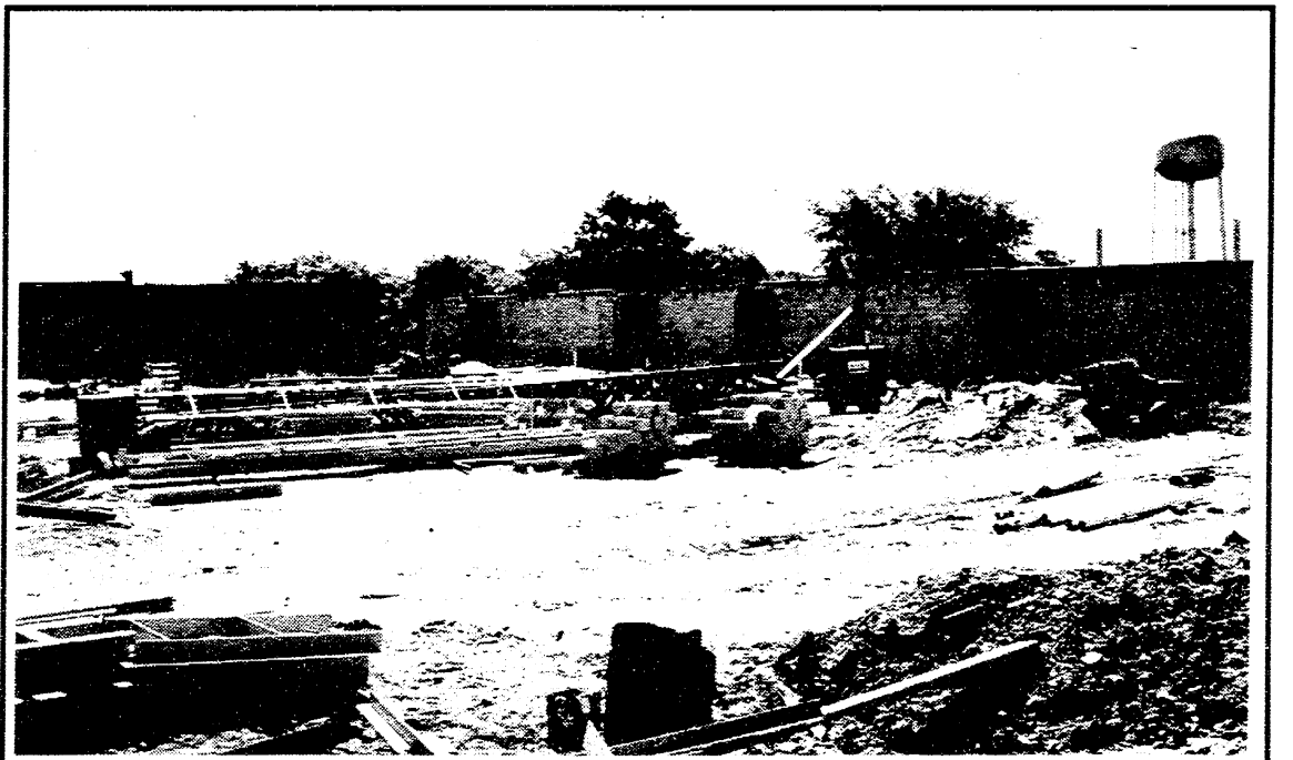
Last week the south classroom walls went up at Klager School.
