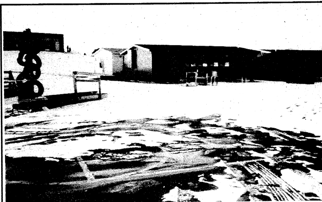
The four portable classrooms at Klager Elementary were moved last week by the "portable specialists" at J.R. Taylor Co. They now sit close to the playground at the east end of the hill.. When the kids return next Monday, they'll find their classrooms ready for learning!
