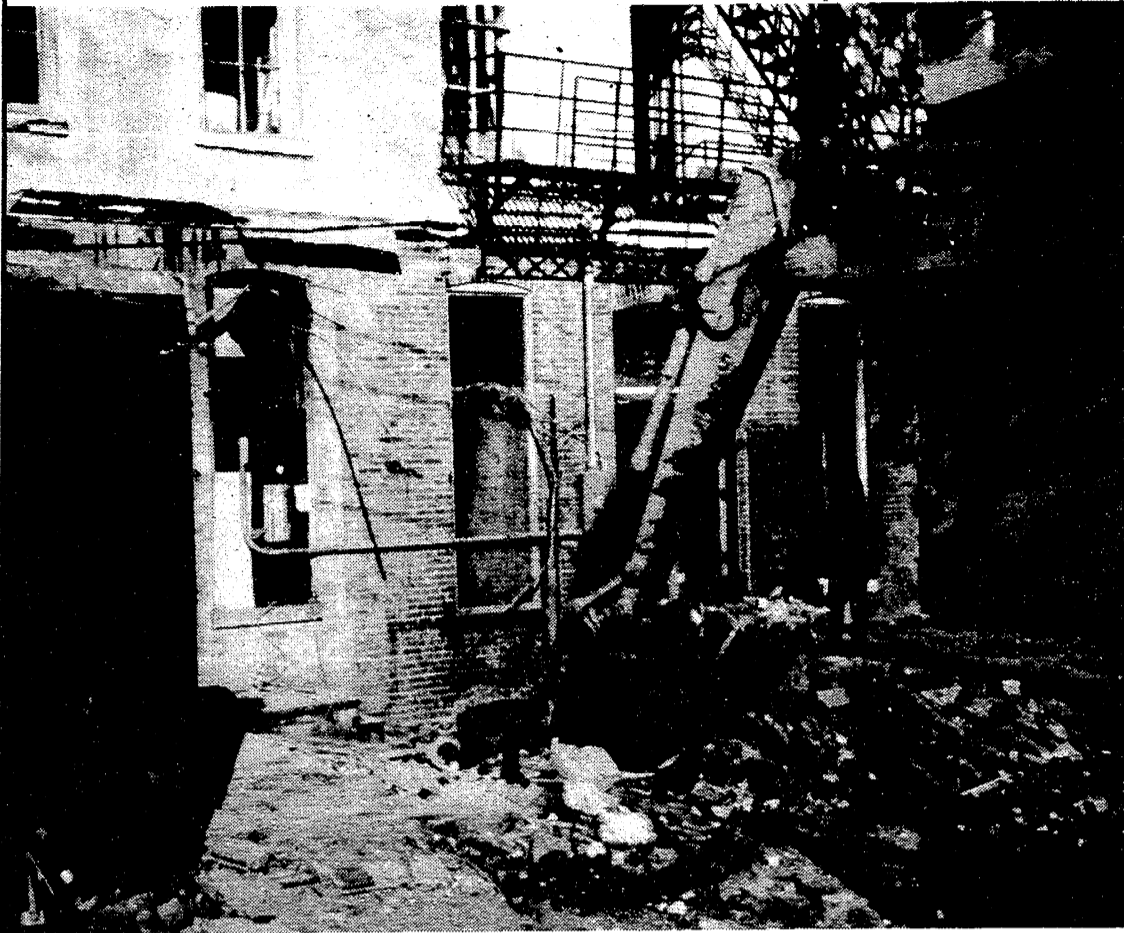
In the continuing work of restoring the old Black Sheep buildings, Tom Ellis, Owner of the Manchester Hotel Building, has begun the process of tearing down the lean-to on the back of the buildings. This shed was not up to current building codes. He has poured footings for an elevator which will service the second and third floor apartments.
