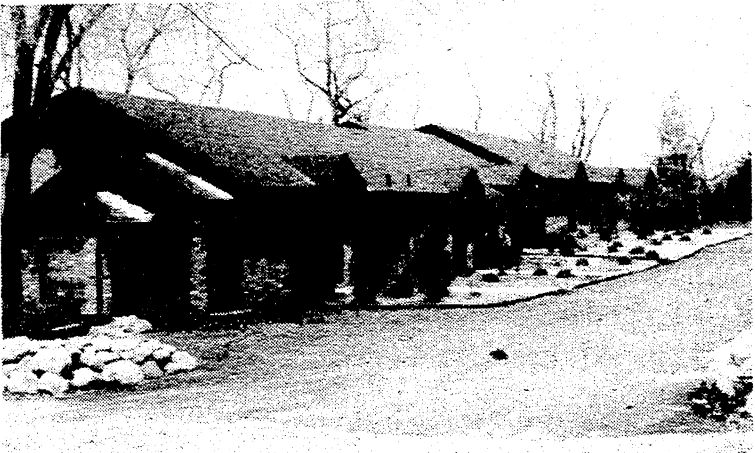
Townhouses on North Washington Street are being renovated as condominiums
