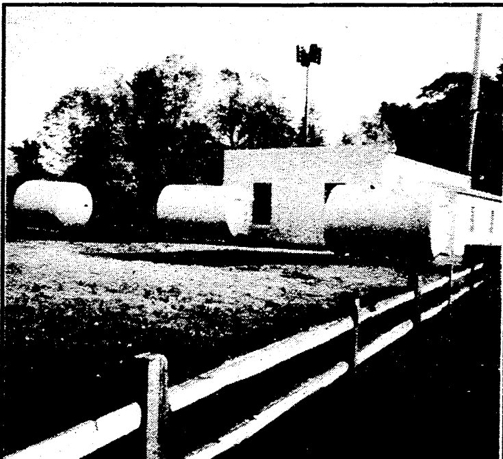
No, this is not new playground equipment at Chi-Bro park! It is part of the new water filtration system which is slated to replace the Village's current (fifty year old!) system this coming November.
