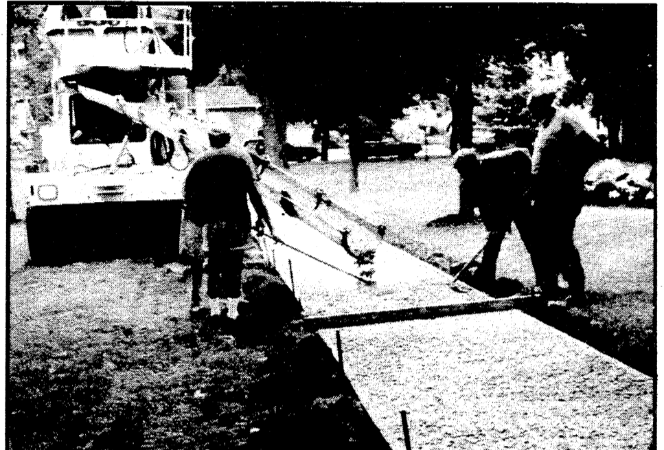
The cement is poured into the framework and work begins. Village Manager Jeff Wallace notes that a garden-type park, which may be the end result of this face-lifting, would be a great addition to our park system.
