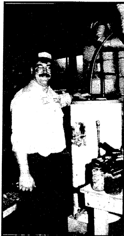
Rick Graustein of Sien Electric rewiring the heater and installing a new electric panel on Kothe Road project.
