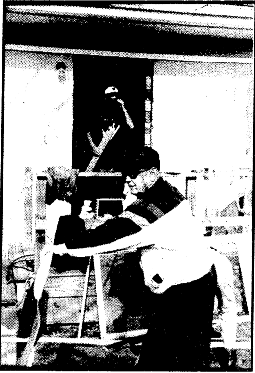
Jerry Ahrens replacing the front door on Hogan Road project
