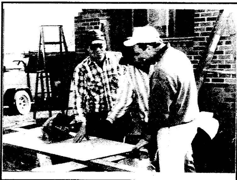
Now here is a crew of Proctor DuRussell and Way with a layout problem while they are reconstructing soffits on Kothe Road.
