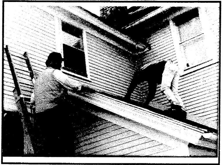
Doug Parr on the ladder assisting Chris Lentz who was doing the work of replacing shingles
