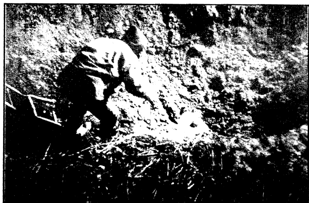
His light provided by floodlight (and not luminarias), Village employee Todd Knepper gets down and dirty on Christmas Eve to repair a broken water main. Also assisting were Brian Kunzelman, Dan Fleck & Jim Wild. Thanks!
