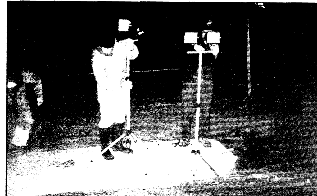
Another example of the best of community spirit is that during the dark hours of Christmas Eve, when most of us were enjoying family time, eggnog, or rest, the DPW and Village Manager Jeff Wallace were out repairing a water main break. These dedicated public servants are also dedicated family people and "just did what they always do" so that the rest of us could comfortably enjoy the holiday.
