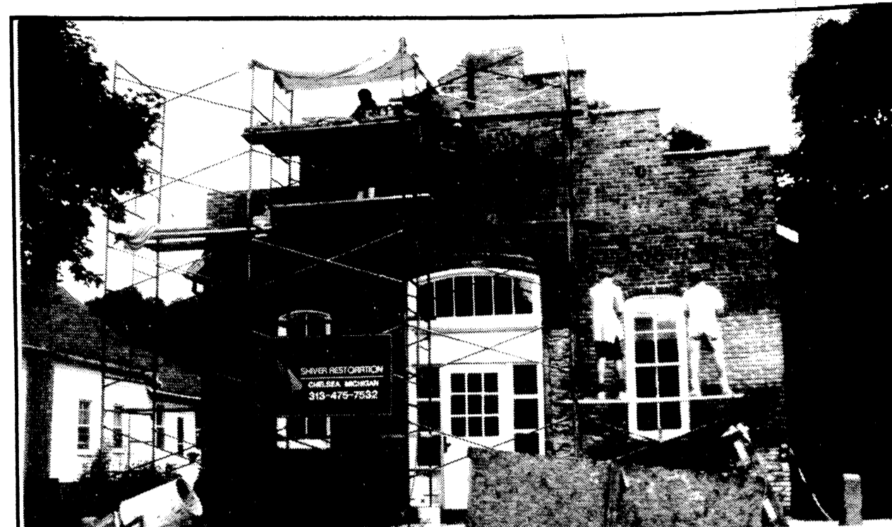
Apparent to even the casual observer on Main Street, the Blacksmith Shop is undergoing a face lift. The roof has been replaced by Mel Sroufe of Mel's Roofing. According to Historical Society Member Reno Feldkamp, Shiver Restoration from Chelsea is also working on brick and window restoration on the building's exterior. "We feel very fortunate to have Shiver's working on our building," said Reno. "They do an excellent job." The work is being financed by a grant from the Chicken Broil as well as proceeds from Historical Society projects (Raffle, Calendar and luminaria).
