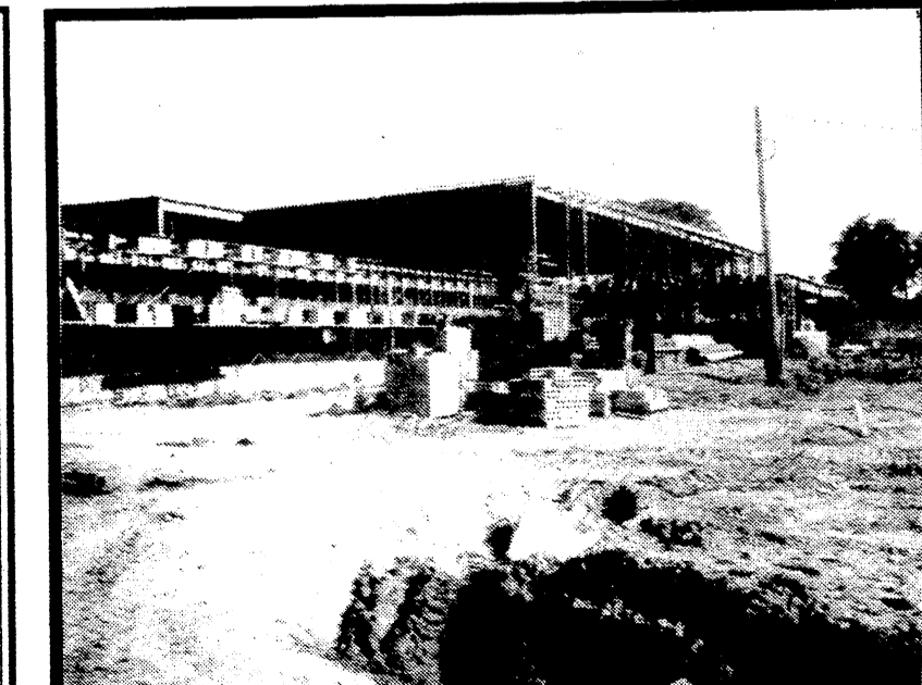
Progress, progress, progress - work is continuing as scheduled at Johnson Controls new R & D facility. See story on Second Front Page.
