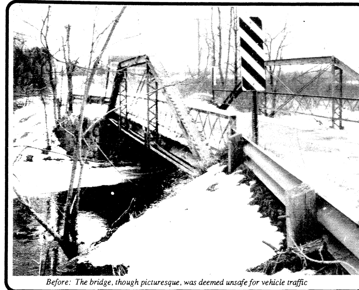
Before: The bridge, though picturesque, was deemed unsafe for vehicle traffic
