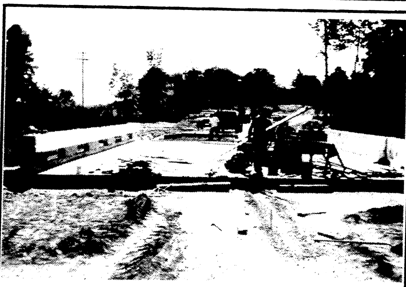
The Allen Road Bridge - "During". Work is completed and the bridge is open to traffic. See Story, Second Front Page
