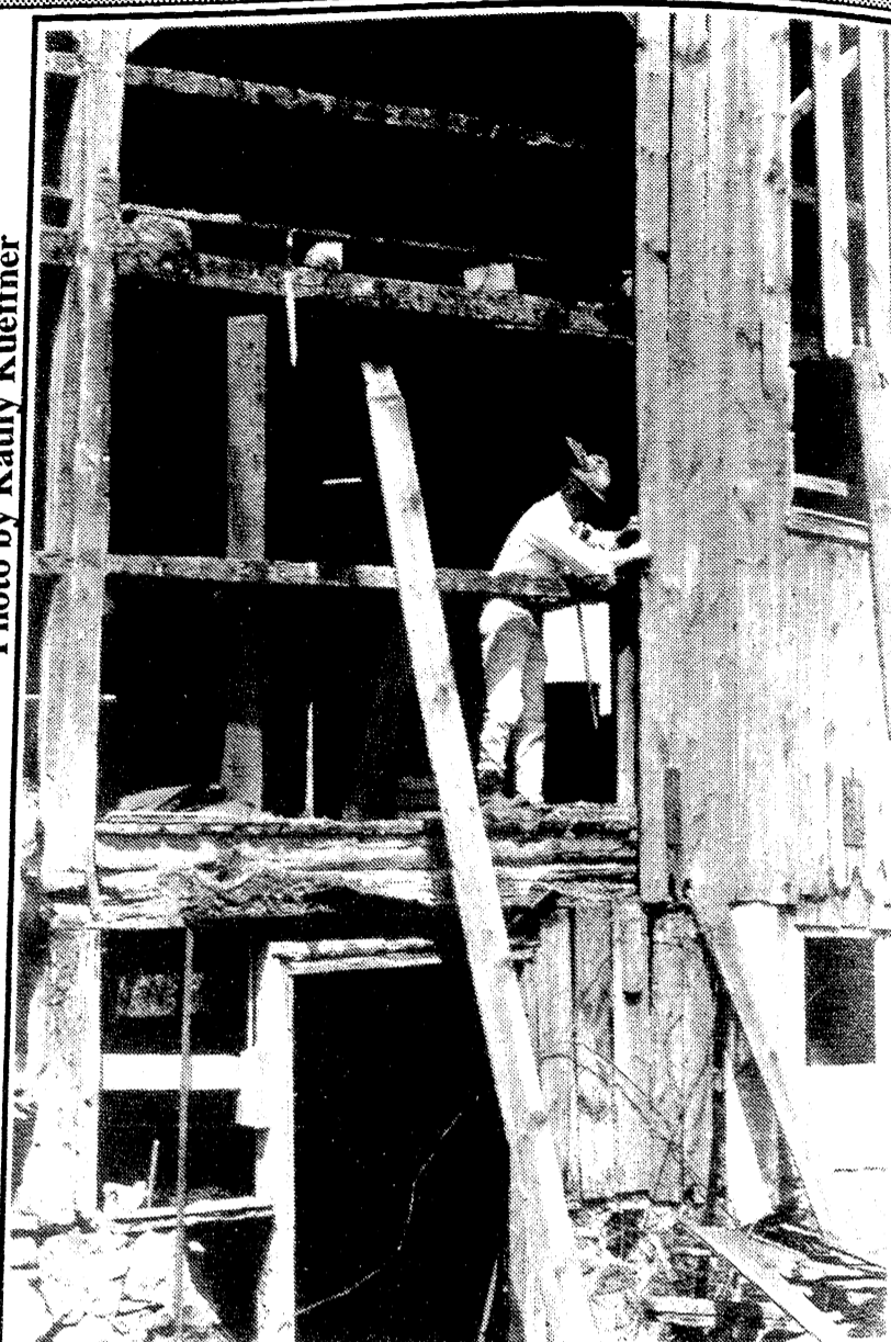
Adjacent to the new Johnson Controls plant site on Parr Road, Don Limpert, pictured above, dismantles and salvages the hip-roof barn built around 1902 by the family of Hiram and Louisa Parr.
