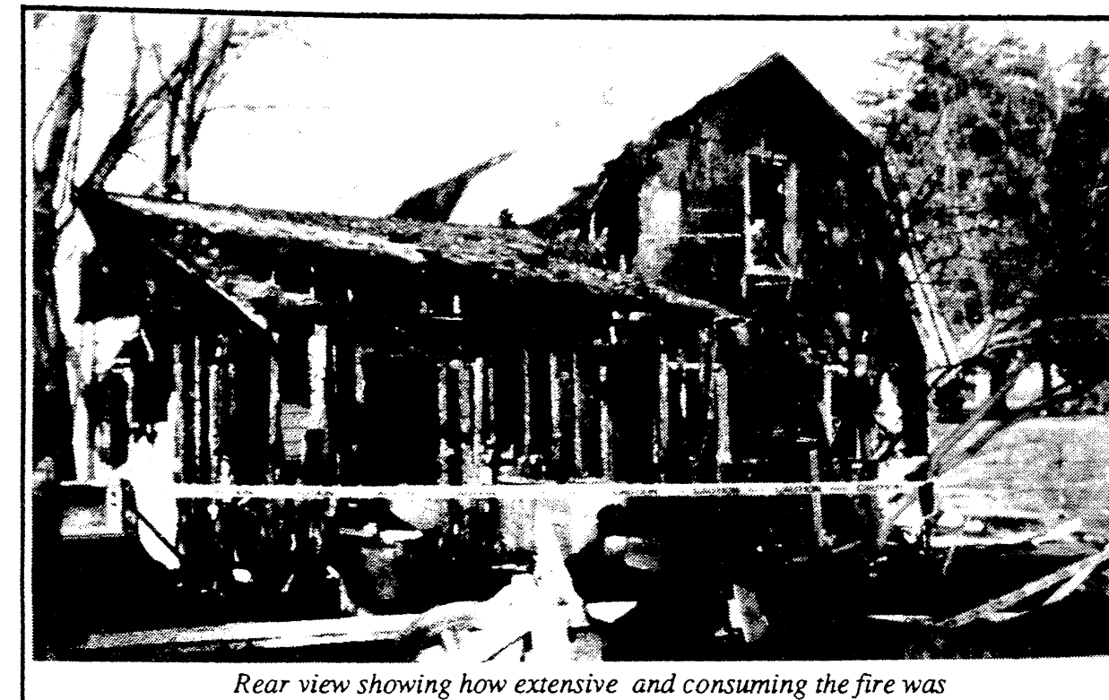
Rear view showing how extensive and consuming the fire was
