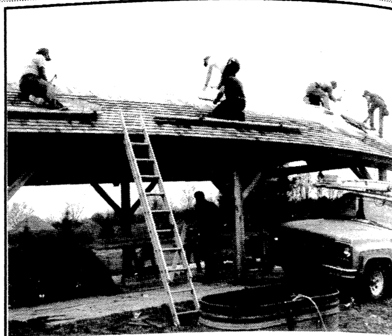
Work on the Men's Club Pavilion in Chi-Bro Park continues. Members pictured above who were shingling the roof: Jerry Ahrens, Scott Mester, R.D. Scott, Pat DuRussel, Mel Shrope and Tom Pratt. - Photo courtesy of Dave Kemner
