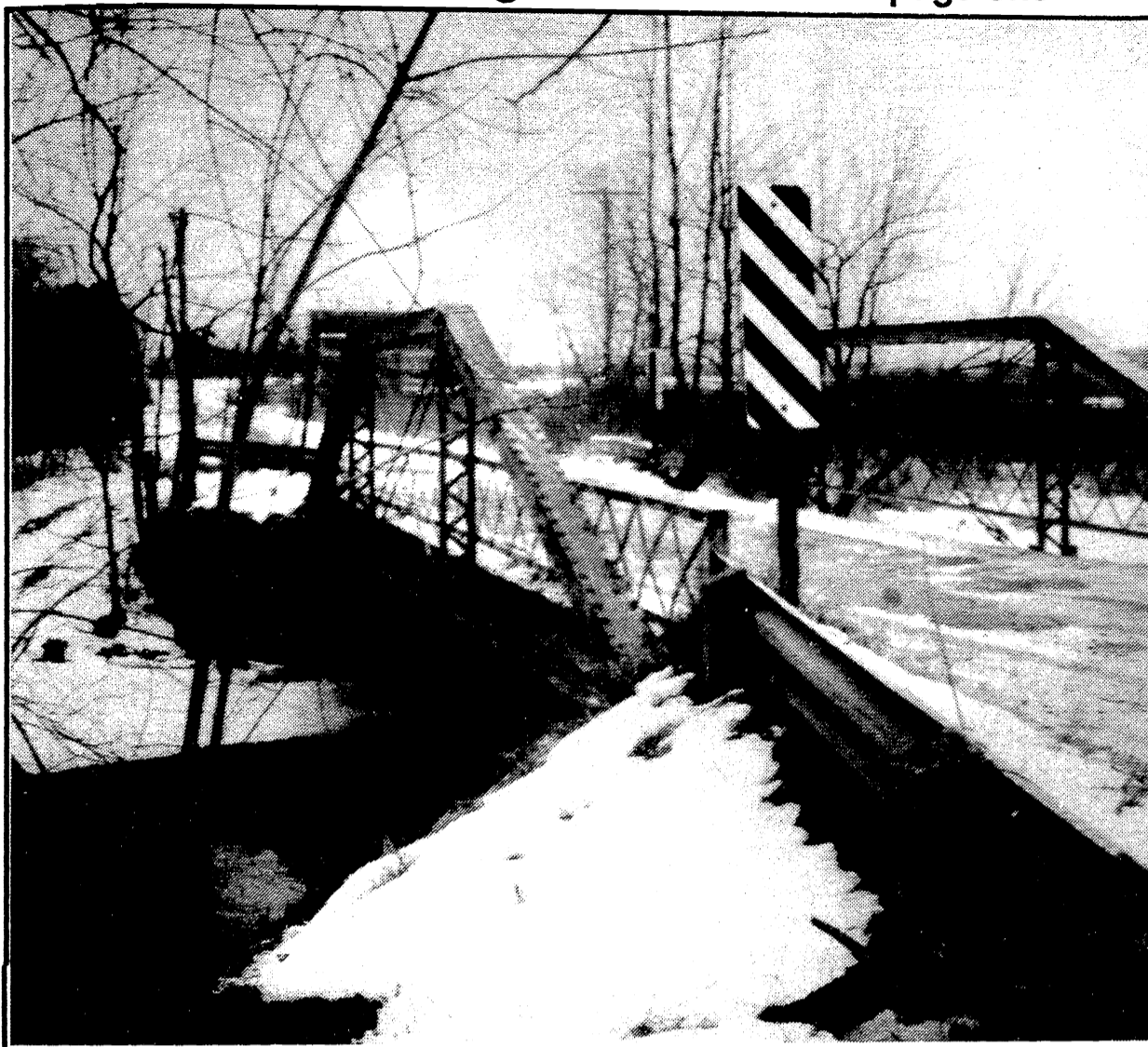
View of the Allen Road bridge. (Photo taken last winter)
