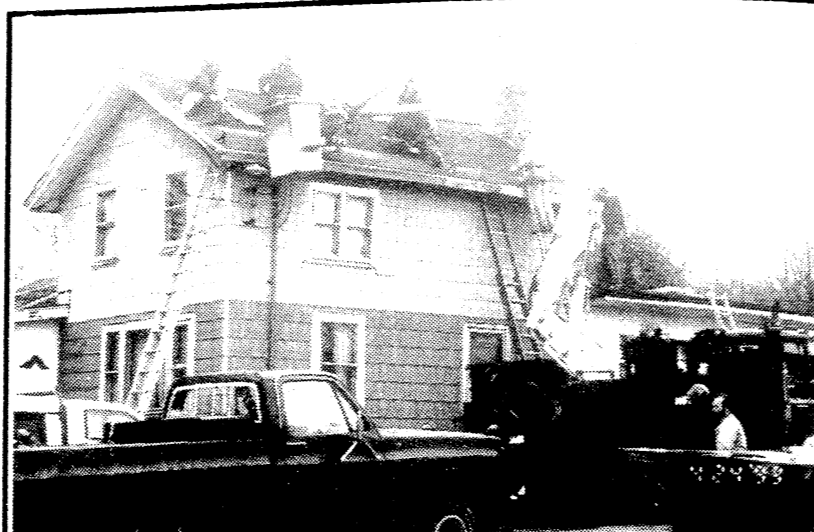
Stein Electric Cherry Picker shown hoisting materials to the roof of Carl Pierson Residence. Missed last week was the house of Laura Gauss on S. Macomb St. See thanks this Edition for additional volunteers names. — EWG
