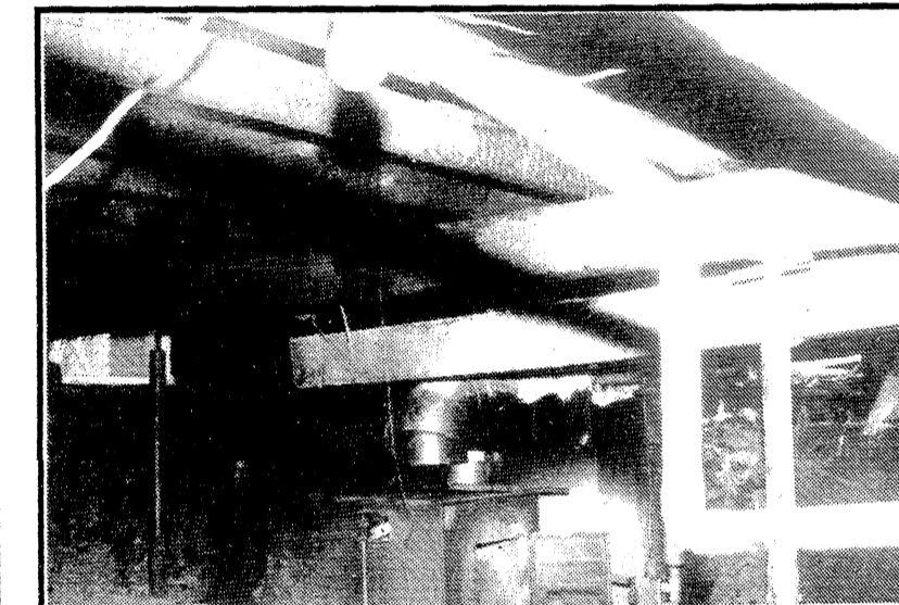
Where fire started, note charred joist, sagging duct's and wire's
