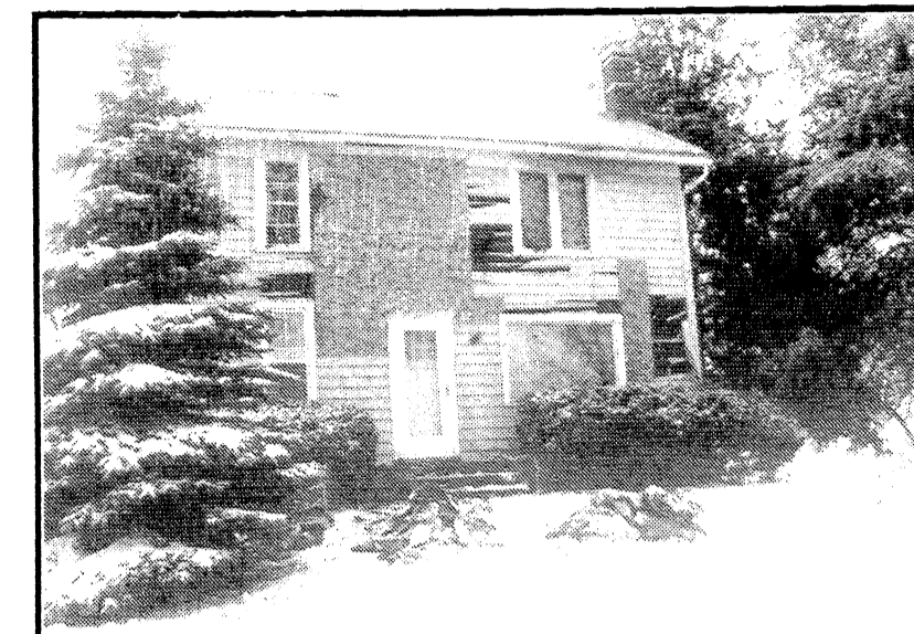
House showing where fire had to be uncovered and extinguished
