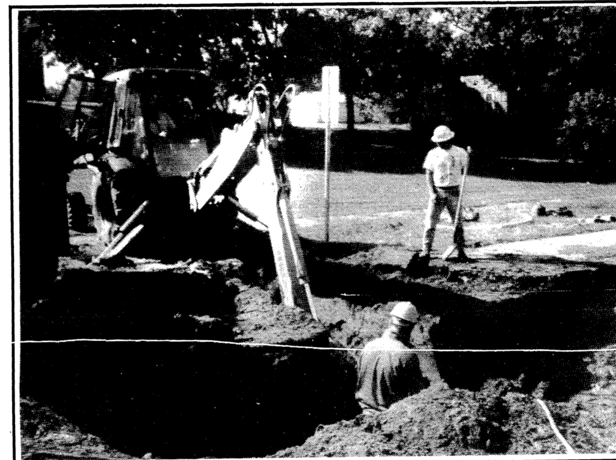
Workmen uncover leak on City Road, 52, between Granger and Furnace
