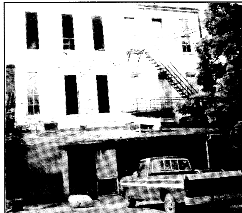
Rear of building, debris cleaned up, note unboarded windows.
