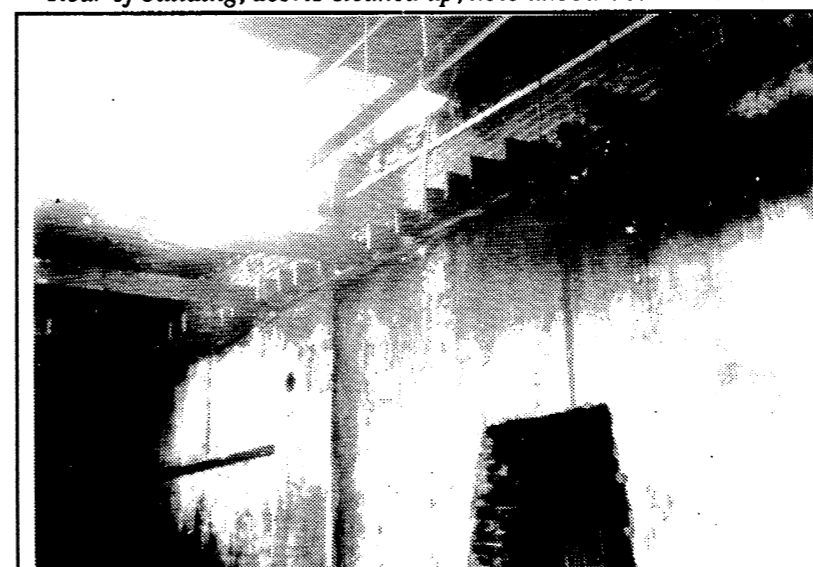
Third floor Ceiling joist cut off and missing roof rafters
