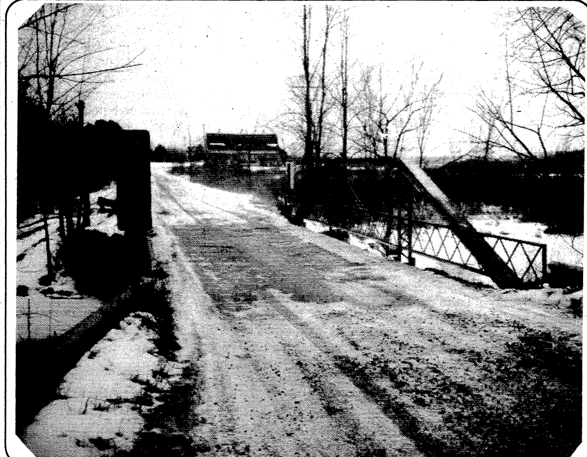
Allen Road is one mile north of Clinton, the bridge is about one half mile west of Clinton - Manchester Rd., Bridgewater Township.
