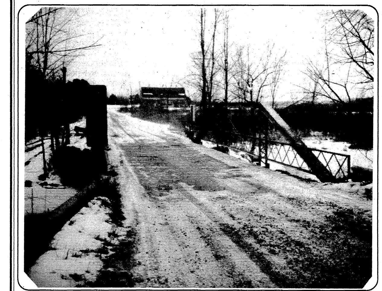
Allen Road is one mile north of Clinton, the bridge is about one half mile west of Clinton - Manchester Rd., Bridgewater Township.
