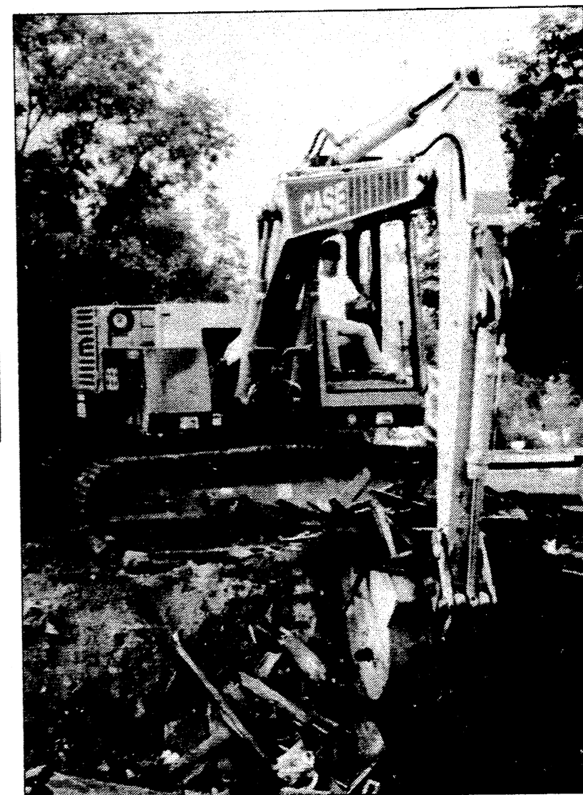
Little Wack Excavating is shown removing left-over debris from a house fire at 202 Auburn that occurred on May 23. The house which belonged to Alma Uphaus has been removed and Ron Milkey said that Premier Contracting Inc. will be building a home for Larry Goodell on that lot scheduled for completion by the end of October.
