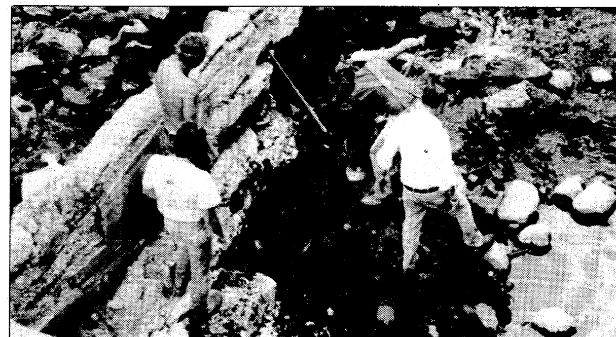
Workers repair the hole in the west training wall of the dam.
