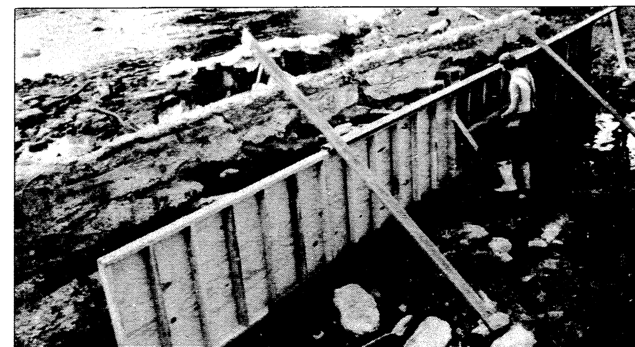
A new wall is being built to replace the deteriorating wall in the background.
