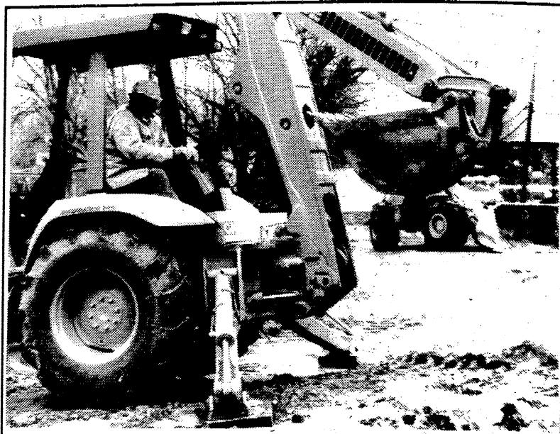
Construction has begun on the sewer separation project in the Village.
