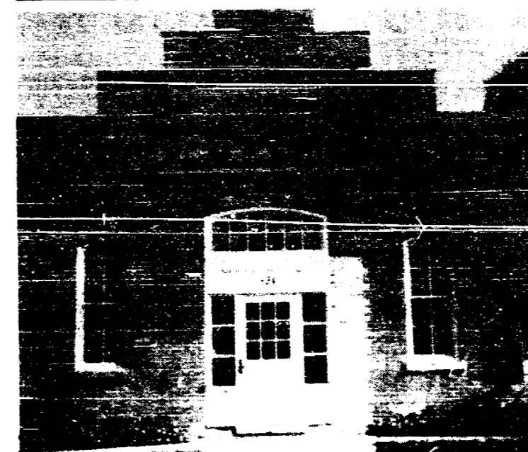
The John F. Schneider Blacksmith Shop. Dedication pictures on page 3
