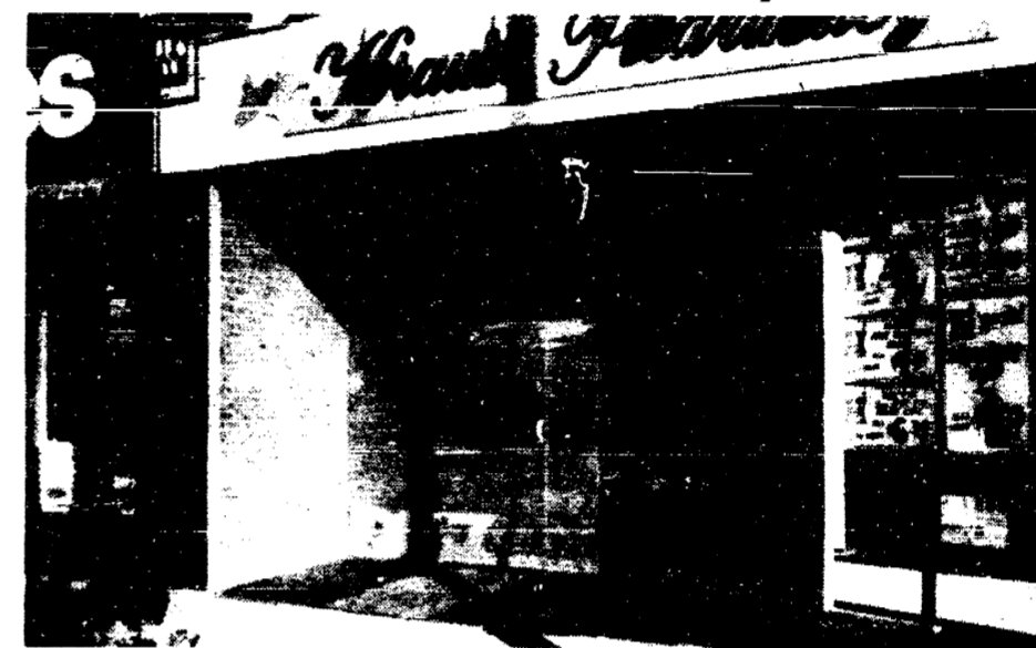
Early Sunday morning, an area driver attempted to back up his vehicle on Main Street when his accelerator stuck making him to smash into the front window of Krauss Pharmacy causing extensive property damage. Krauss Pharmacy is asking its customers to please use the back entrance of the store and is very sorry for the inconvenience.
