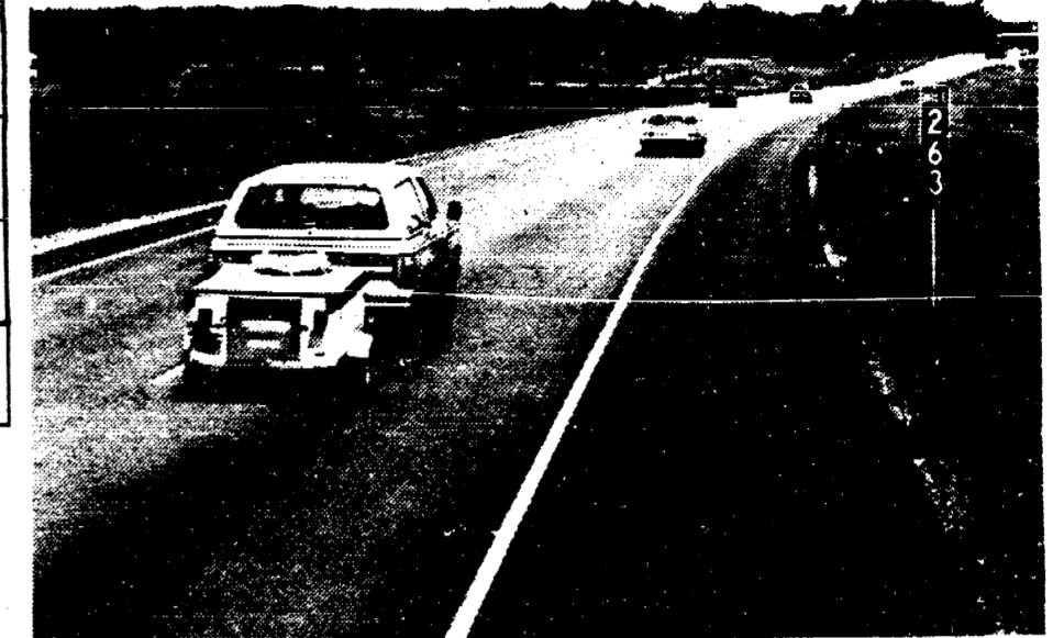
NOT AS YOUNG AS SHE LOOKS -This stretch of I-75 freeway north of Graying has had a face lift that makes it look brand new even though it's more than 20 years old. It is one of many Michigan highways that have undergone recycling, a process that involves tearing up the roadway, mixing the pulverized material with a quantity of new asphalt and laying it back down. The result is a good-as-new highway at a saving in cost and materials.
