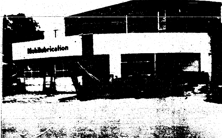
Demolition of Mobil Gas Station at the corner of M52 and Main Street in the Village of Manchester, commenced Tuesday, September 2. Owned by McPherson Oil Company of Howell, Michigan, the building had deteriorated past repair.
