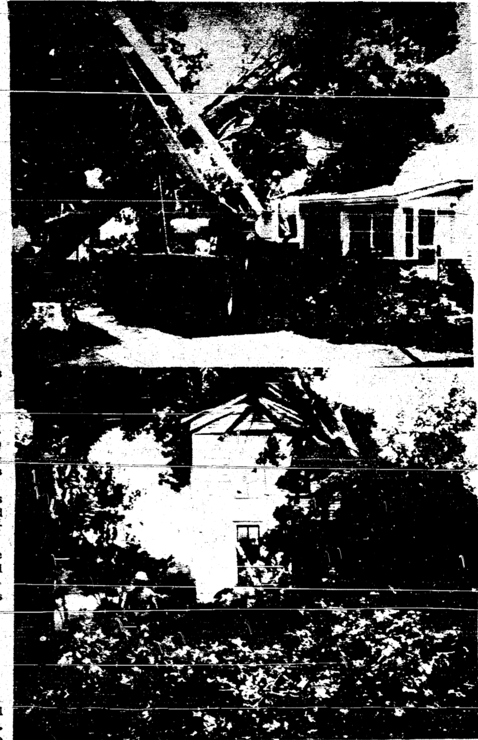
Sunday's storm did considerable damage to the home of Mrs. Lavon Hudkins of 327 South Macomb Street. A large maple tree fell into the front of the house, roof and gable. The damage was estimated to be $2500.
