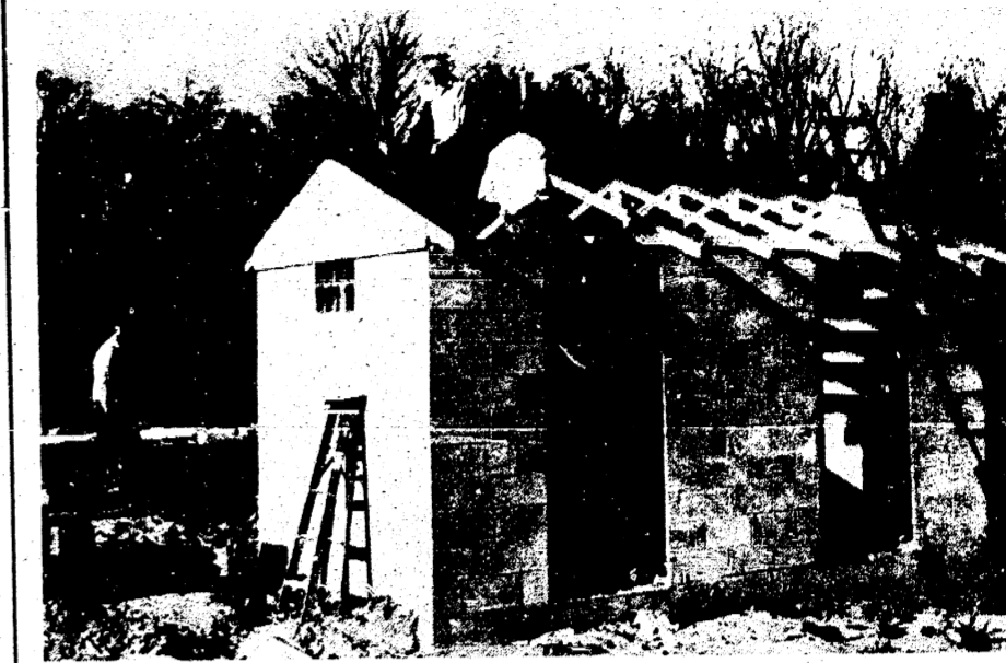
The Jaycees of Manchester putting the roof on the restrooms at Kirk Park. This is only one of the many community projects that they sponsor throughout the year. Pictured are Ron Panches, Jim Hartman and Bill Panches. Picture by J. Morton.
