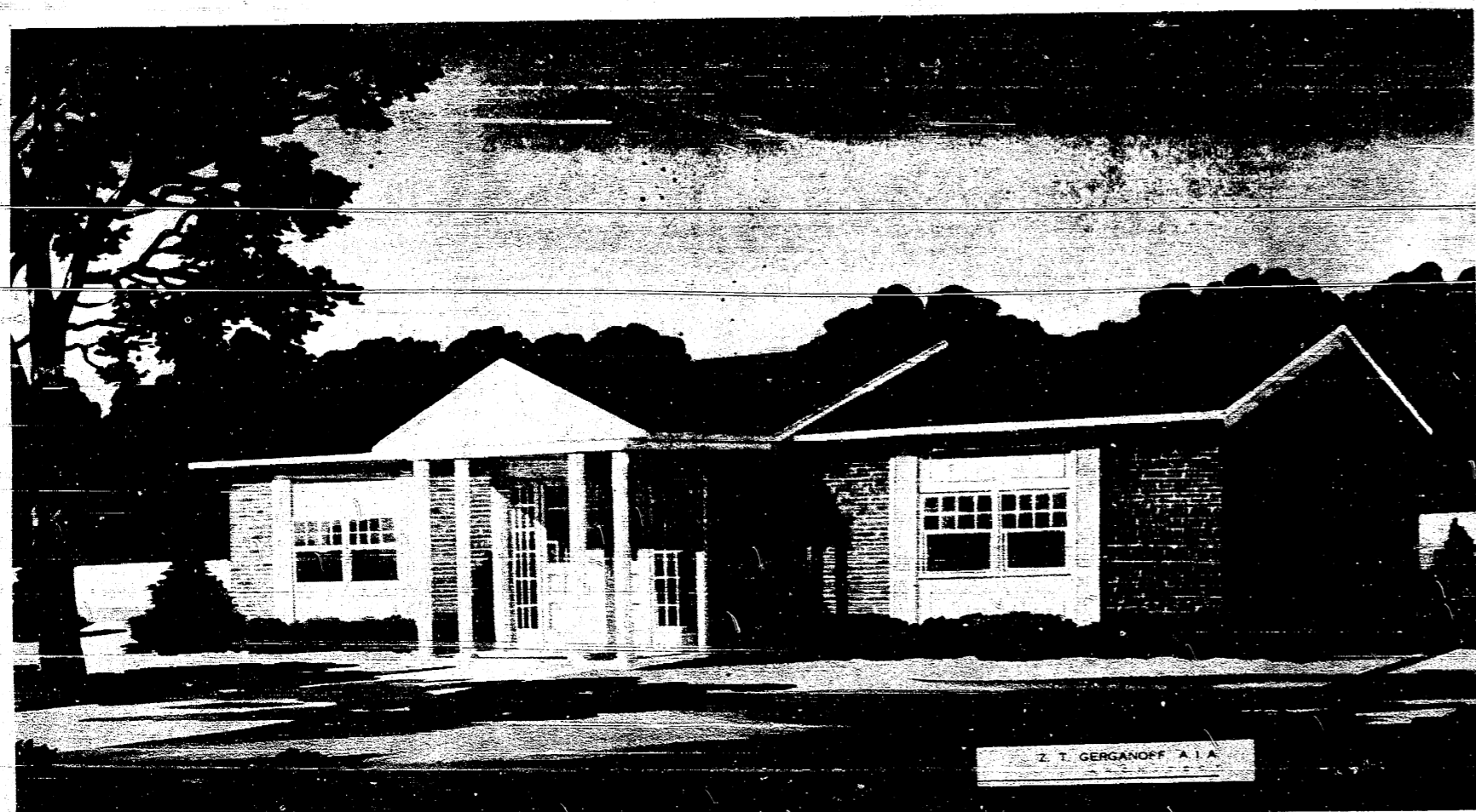
NEW SALINE OFFICE AT 179 E. MICHIGAN AVENUE, NEAR HARRIS, IN SALINE
