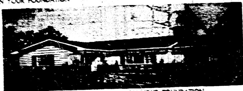
COMPLETE and ERECTED ON YOUR FOUNDATION
