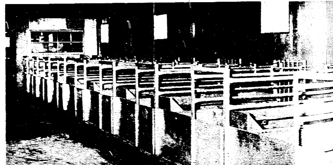
There are 20 farrowing stalls in the front half of the building, 10 on a side. The rear section of the building is occupied by 10 weaning stalls. A radiant heating system in the floor insures that the pigs are comfortable on the coldest days.
