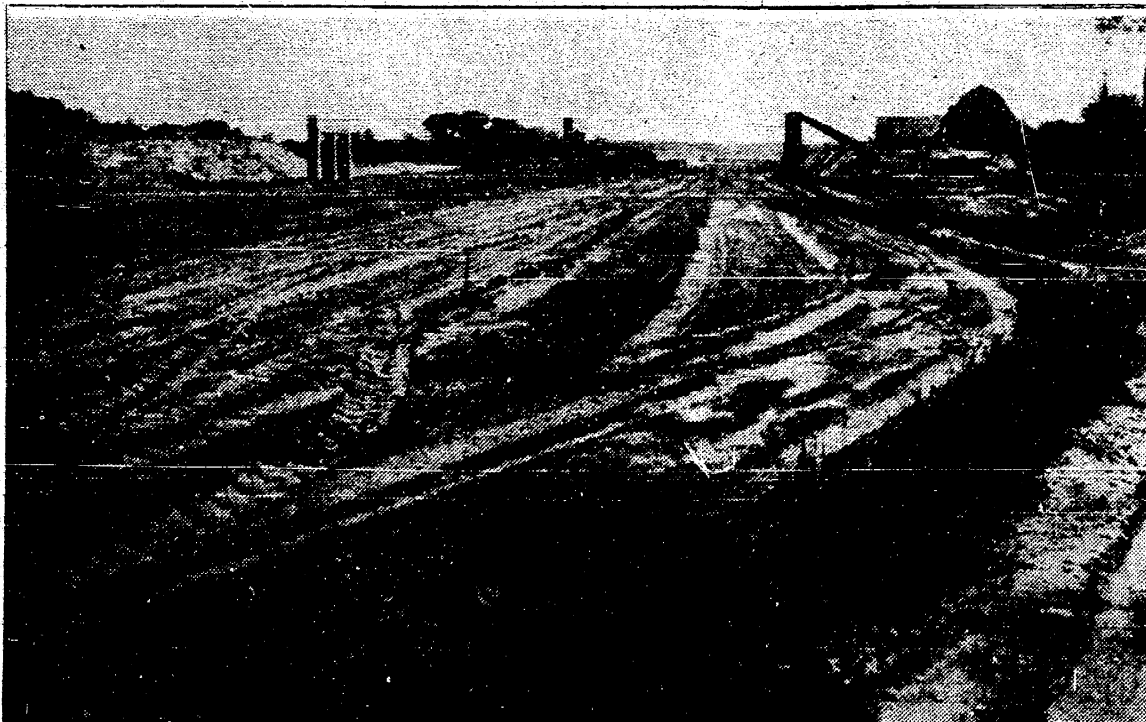
HIGHWAY WORK PROGRESSES: Work is progressing on construction of the US-12 expressway near Chelsea. Grading and bridge construction shown here is near Silver's restaurant in Lima township. The route will become Interstate 94.
