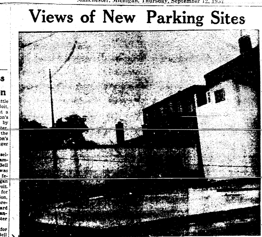
SPACE FOR THE NEW Union Savings Bank parking lot is shown as it nears realization following the demolition of the building which formerly occupied the spot. The lot is located on Adrian Street, one block south of Main.
