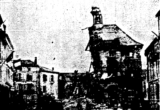
One of the freak effects sometimes achieved by high explosive bombs is seen in this photo of a town in Finland, on the U. S. Third Army front. The big building at the end of the street took a direct hit and rubble, the other remained standing firm.
