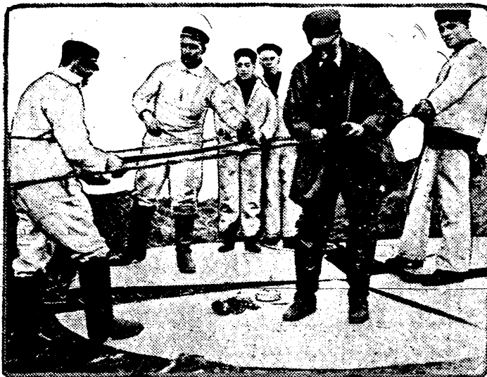
INSULATING NEW CABLE
