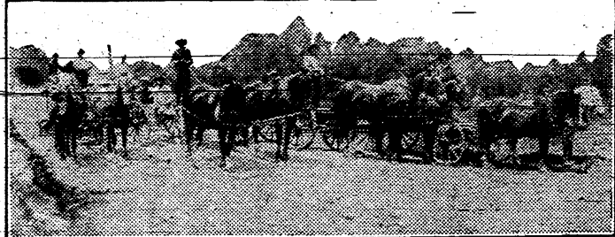
Road Building in Emmet County.
