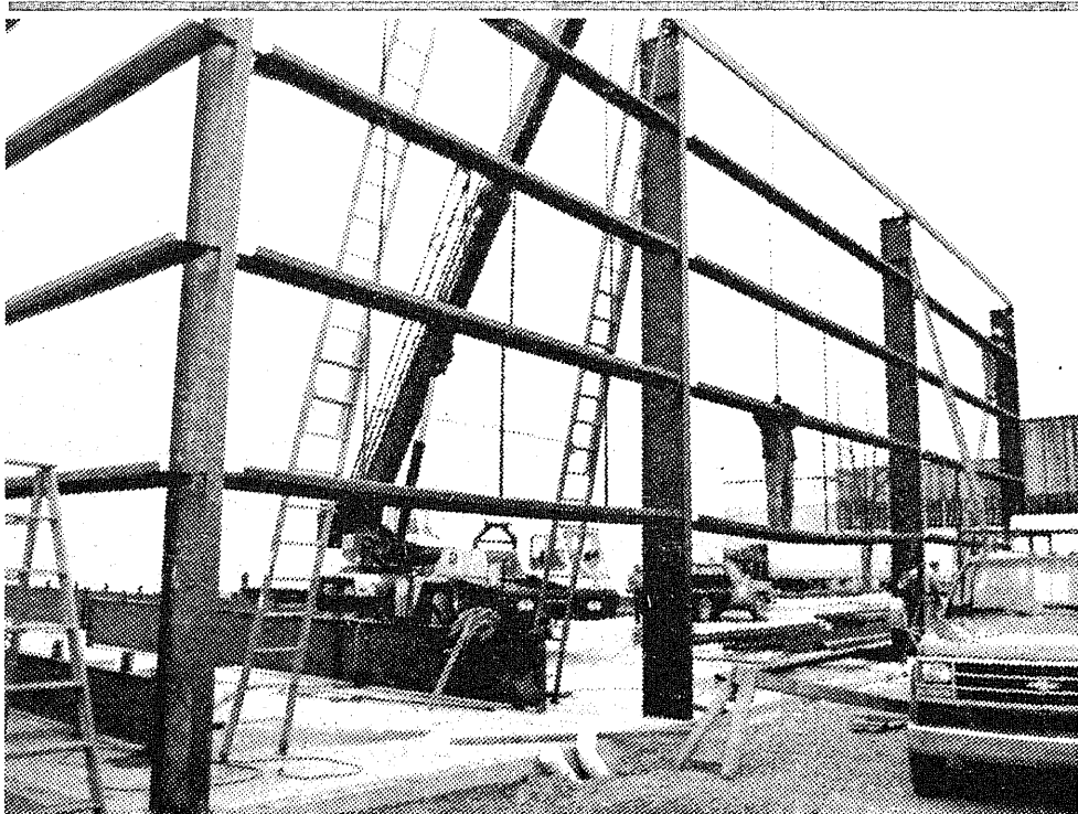
SEBEWAING INDUSTRIES IS GETTING some more elbow room. The company is expanding its warehouse on Albert Street with an addition of 100 x 190 feet because more room is needed to store parts, said Plant Manager John Meininger. The $179,000 addition is being built by Sobczak Construction of Bad Axe is doing the work. Completion is expected in about two weeks. MARY DRIER PHOTO
