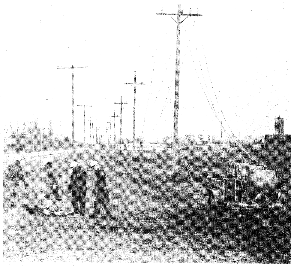
MORE POWER TO YOU: Detroit Edison workers add more transmission lines in the Pigeon area to keep up with a growing demand for electricity by residents and industry.
