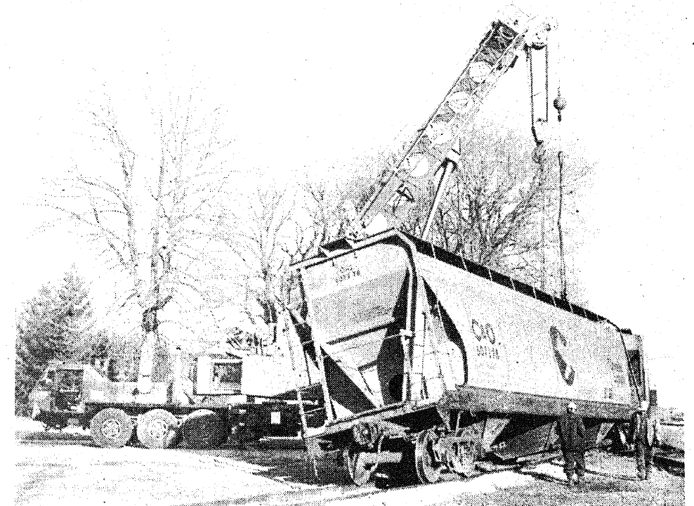
DE-RAILED: Two C & O Railroad grain cars required a boost from a crane to get back on track last Thursday. Softened soil from spring thaws under the tracks on a siding used by Co-op Elevator in Pigeon is believed to be the cause of the cars jumping the tracks. Both cars were loaded with wheat at the time, with each car representing about 130 tons. RICH SWARTZENDRUBER PHOTO
