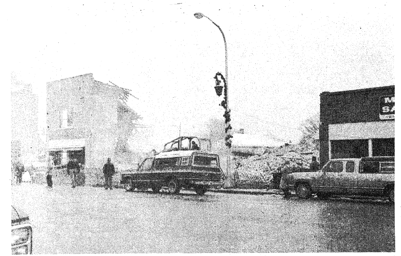
THE OLD BUILDING goes DOWN, DOWN, DOWN in December, 1984, prior to starting construction in Spring of 1985.
