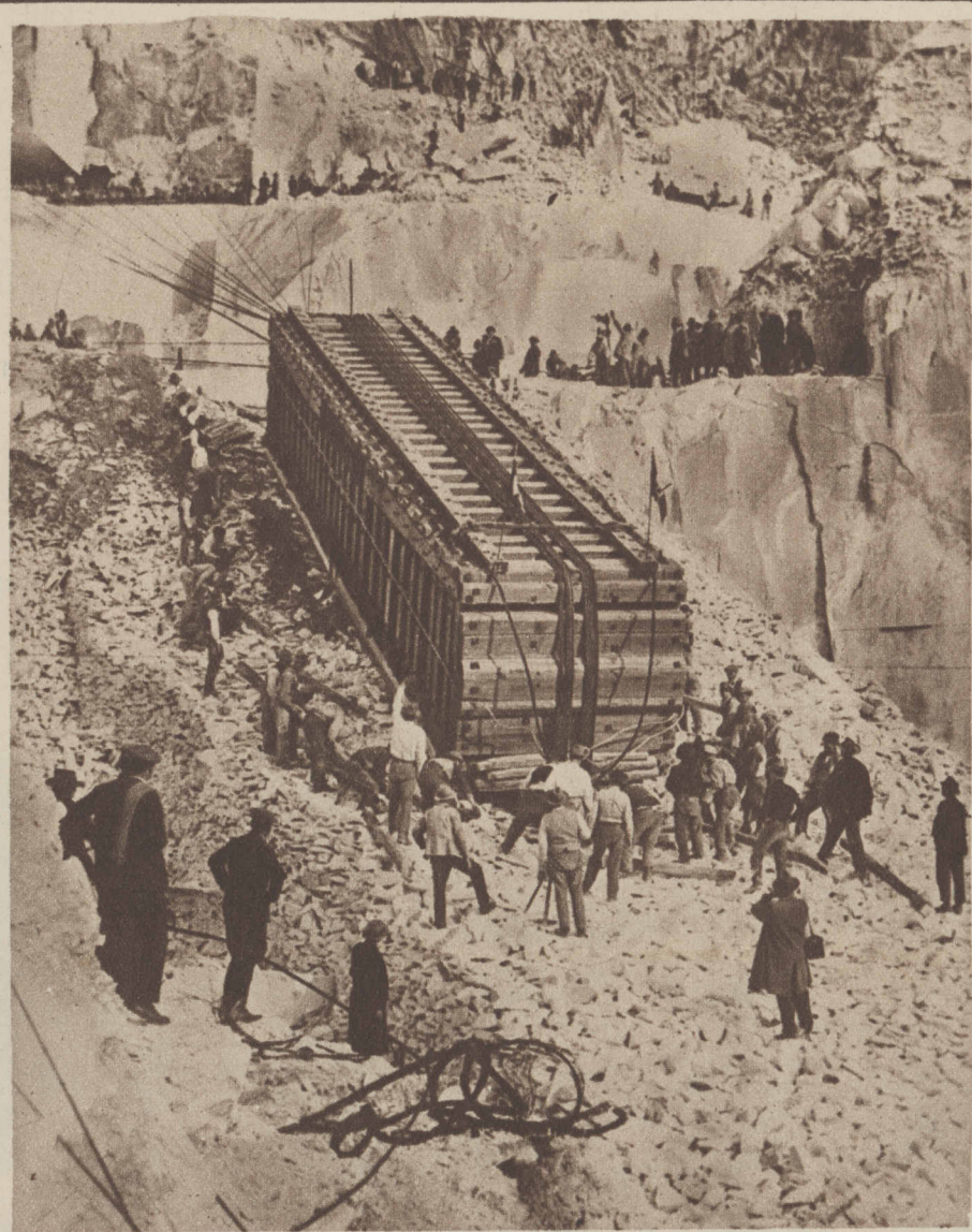
FIFTY TONS OF MARBLE, the largest block on record, was carved out of the quarries at Carrara, Italy; slid down the mountain-side, and started on its way to Rome. There it will be cut as an obelisk to be placed in front of the Mussolini stadium. (Photograph from Wide World.)
