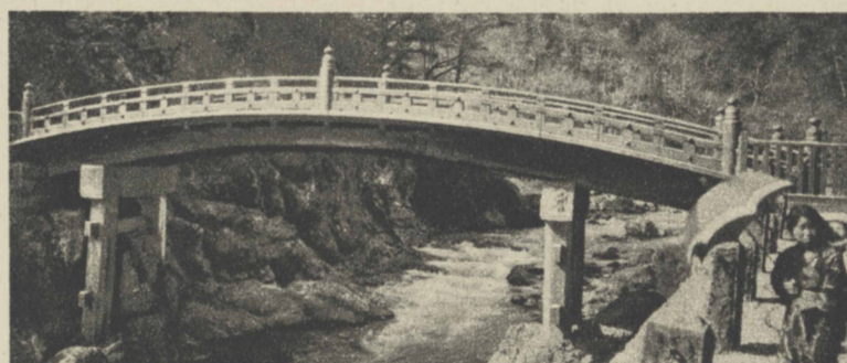
(Ewing Galloway photo.) The ancient Red Lacquer bridge of Nikko, Japan, is slightly arched, but in principle is an independent-span bridge.
