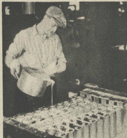
6 From great 3,000-pound kettles the catalin is drawn off in ladles and poured by hand into the molds, where it hardens quickly.
