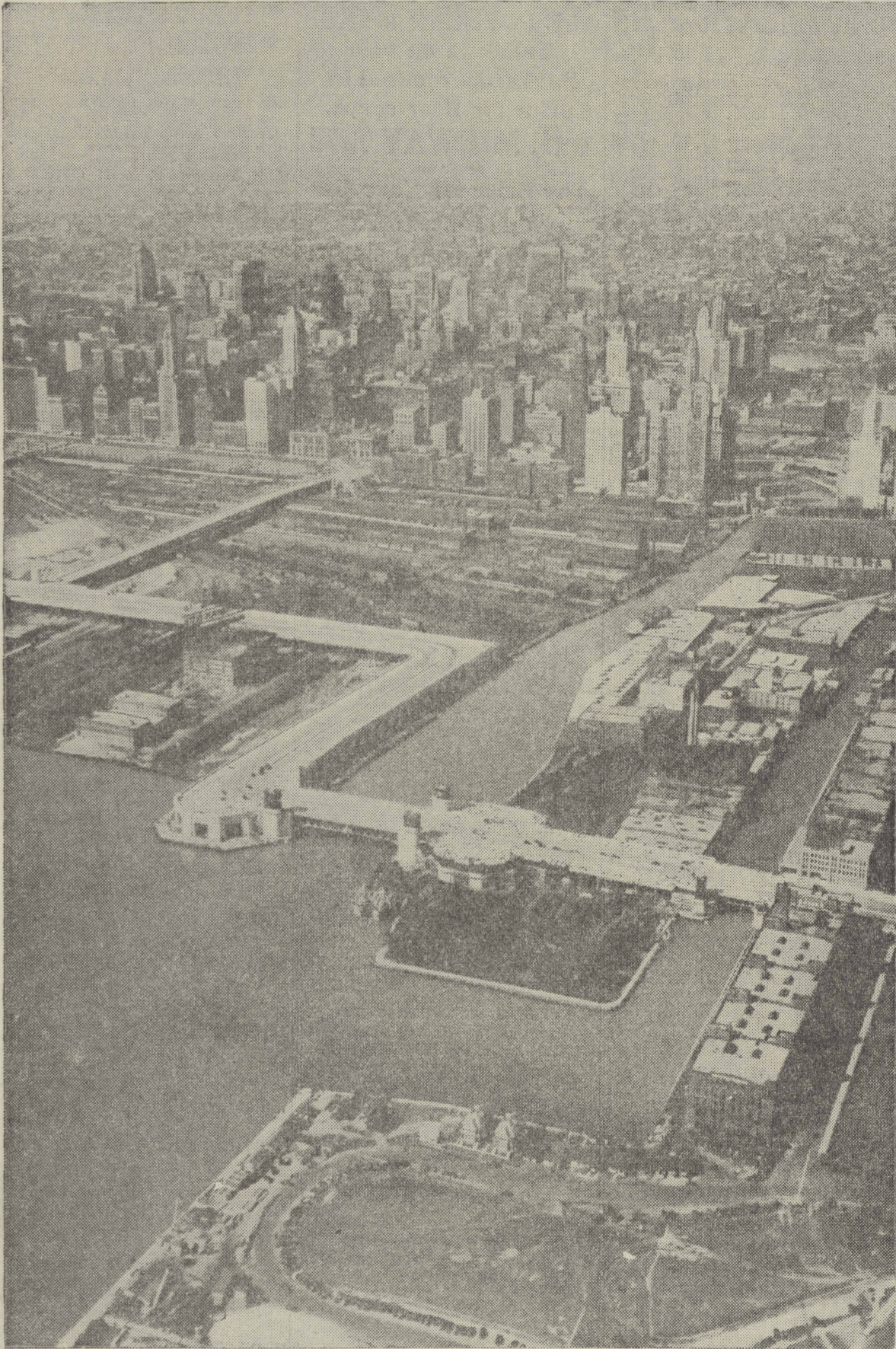
NEW BRIDGE AND ITS APPROACHES —Aerial photo of Chicago's new outer drive link bridge and span over Ogden slip (at right), which will be dedicated tomorrow, with approaching driveways from north and south. One hundred thousand autos are expected to cross the bridge on dedication day.
