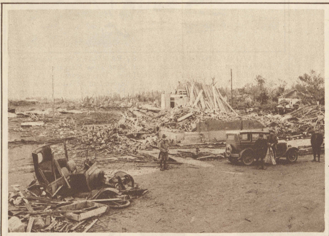
AT DAVIS, SOUTH DAKOTA, troopers guarded the wreckage of the post-office, following the storm which resulted in fourteen deaths and property loss of more than a million dollars in Nebraska, South Dakota, and Iowa. Half the buildings in Davis were destroyed.
