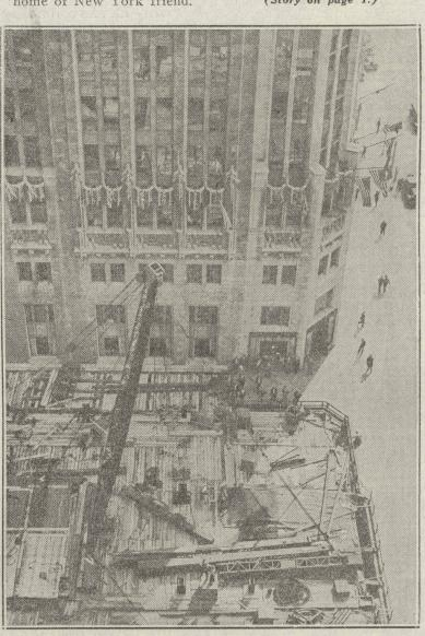
ERECT DERRICK FOR WORK ON W-G-N STUDIO. View from the 15th floor of the Medinah club showing workmen swinging derrick into place at site of radio station just (Story on page 23.) north of The Tribune Tower.
